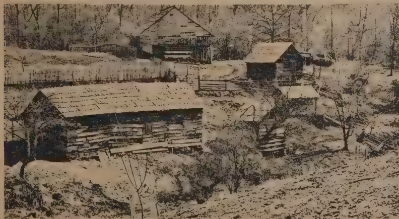
WILLIE GIBBONS FARM — Willie Gibbons, an in-law of the Hensleys, lived on this farm that is currently under restoration. Gibbons' 22' x 45' cabin is at left followed by (from left) a smoke house, chicken house, granary and a barn (background). The barn measures 29' x 40' and has individual stalls for the animals and a full-sized loft.
